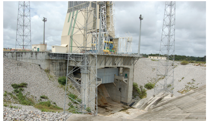
Figure 16 – Cross section geometry of the pylon installation on the Soyuz LPS and picture of the flue (flame exhaust)
